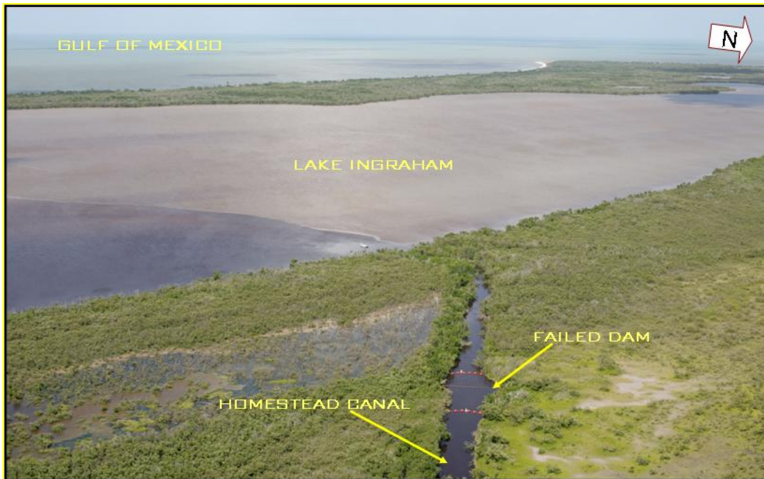
Figure 1.3 – Aerial View of Homestead Canal Failed Dam
