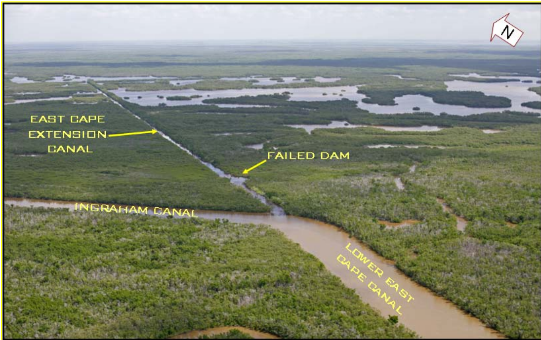
Figure 1.2 – Aerial View of East Cape Extension Canal Failed Dam
